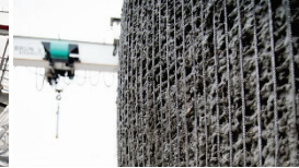
3D Printed steel mesh later filled with concrete, ETH Zurich
