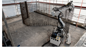
3D Printed steel mesh later filled with concrete, ETH Zurich
