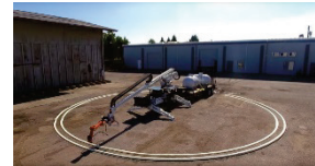
3D Printed building from foam using on-site material, MIT
